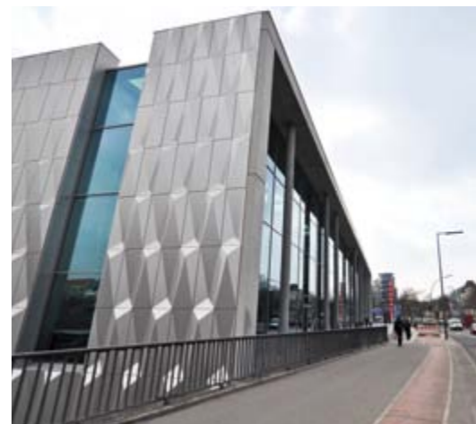
Bauhaus building centre – Berlin, GER
